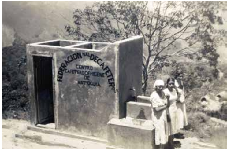
“Rural aqueduct of “La Loma”, municipality of Fredonia”, Antioquia, 1940’s. Construction of water collection and distribution tanks; water pipe network and water facilities; two public showers and sinks that benefit 36 houses. The people involved in the project contributed $281,50 pesos for materials and the FNC contributed $5,828.21 pesos for materials and labor. Sanitation Campaign, Photography Album, p. 1. Photographic Archive, Departmental Committee of Coffee Growers of Antioquia.
