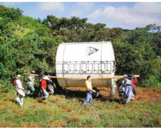
Construction of the aqueduct in Nazareth county subdivision, El Retiro, Antioquia, 2006. Photographic Archive, Departmental Committee of Coffee Growers of Antioquia.
